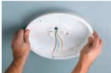
Attach to the housing on the centre plate by rotating.
