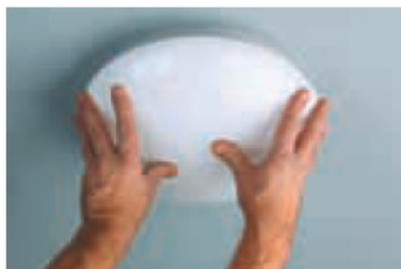
Finally, fix the diffuser in place.
