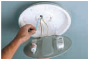
Connect the wires to the connectors.
